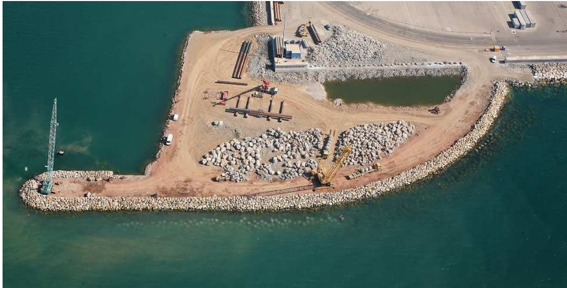
Figure 11. Aerial view of the San Andrés breakwater under construction.
