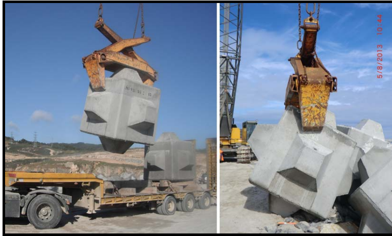
Figure 8. Single pressure clamps handling and placing Cubipod units on the armor slope.
