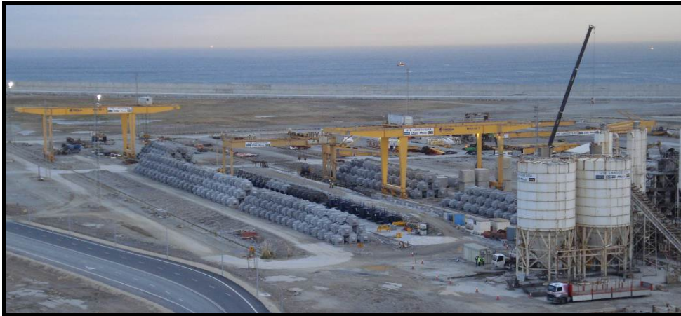
Figure 6. Block yard, gantry cranes and stacking of 15-tonne and 25-tonne Cubipod units in three levels.
