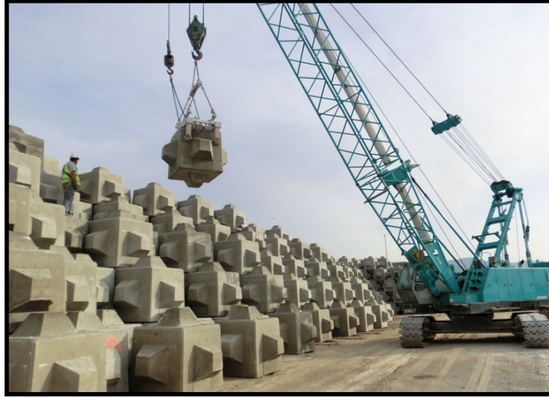
Figure 1. Cubipod CAUs stacked in the block yard (Port of Málaga, Spain).
