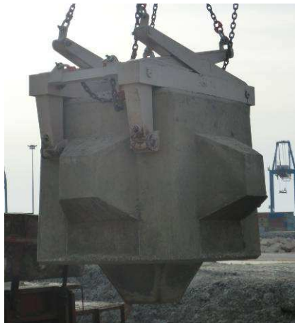
Figure 1. Cubipod CAU handled with pressure clamps.
