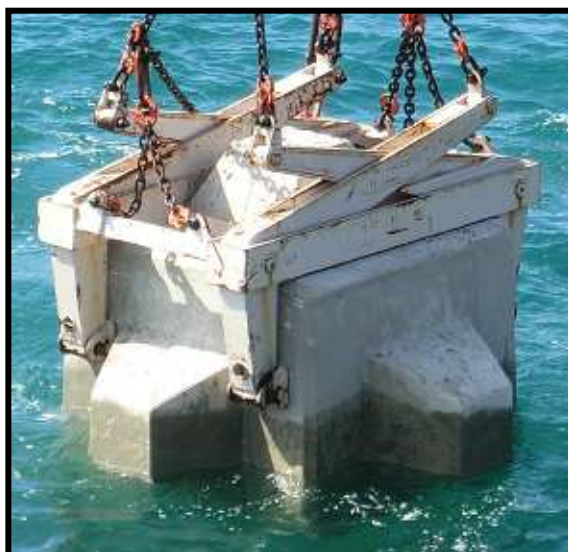
Figure 1. Double-pressure clamps handling a Cubipod armor unit.
