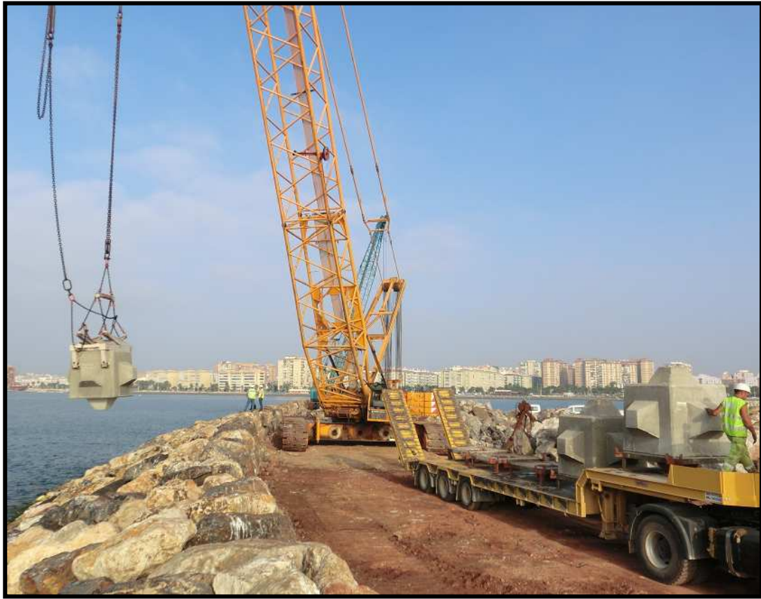
Figure 8. 6-tonne Cubipod armor placement in San Andrés breakwater.
