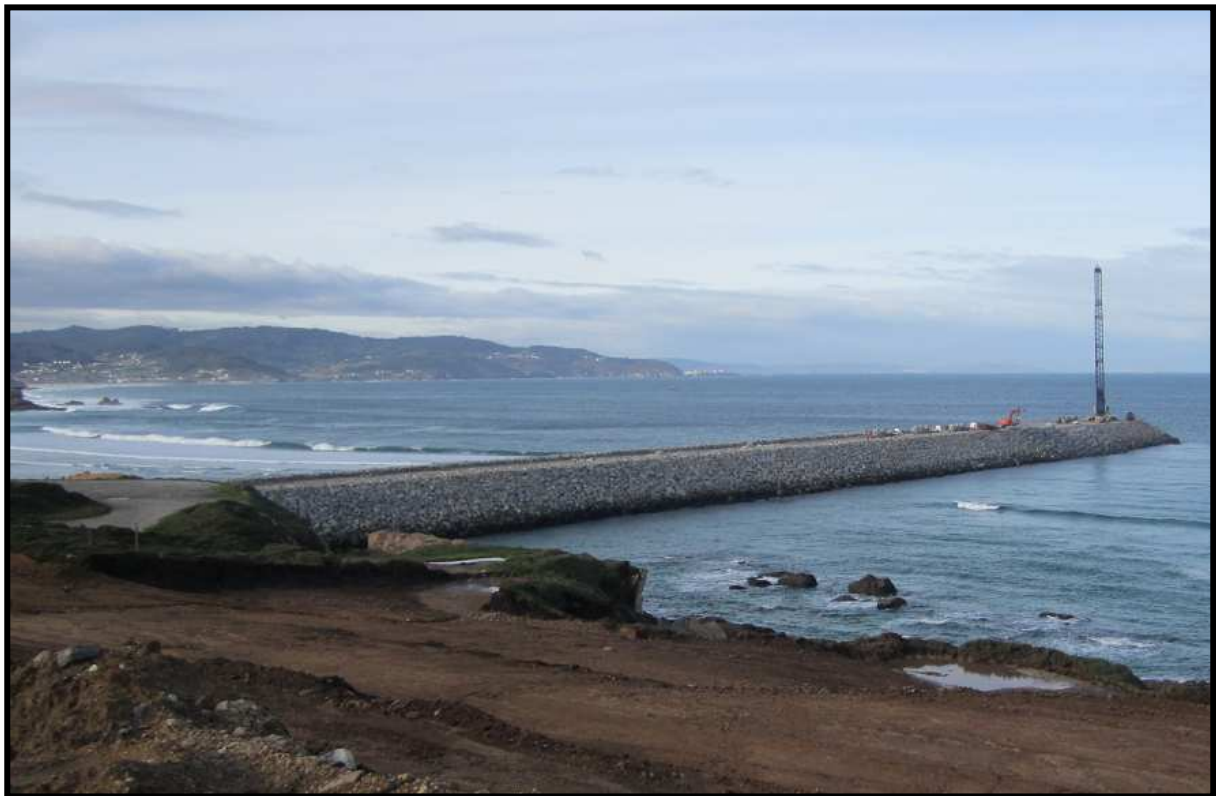
Figure 9. 25-tonne and 15-tonne Cubipod armor unit placement in Punta Langosteira.
