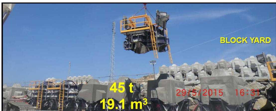
Figure 9. Vertical formwork moving to a new base in the block yard.
