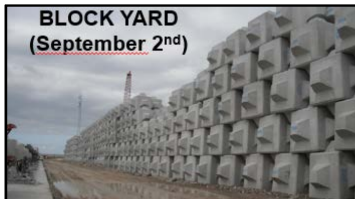
Figure 8. 25-tonne Cubipods stacked in five levels in the block yard.
